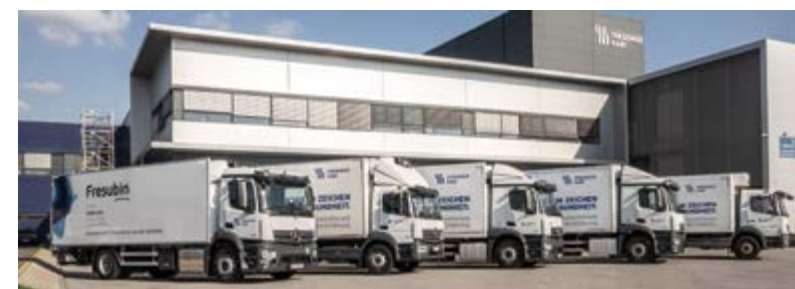
Das moderne Cargo-Center in Werndorf
