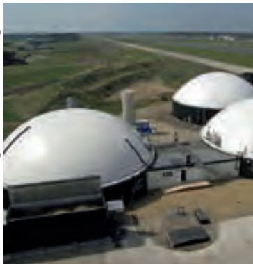
Biogas Plant, Suffolk, England
